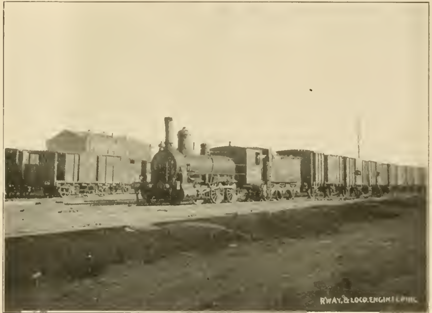
A RUSSIAN FREIGHT TRAIN. ENGINE BUILT IN GERMANY. CARS CONVERTIBLE SO AS TO CARRY SOLDIERS IN WAR TIMES.
